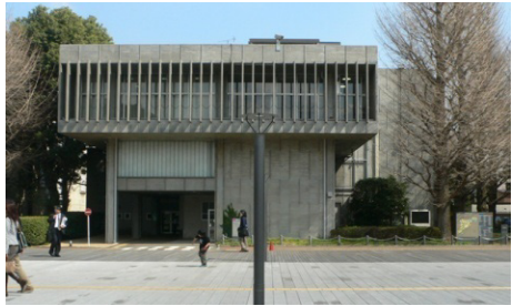
Administration Bureau No. 1 1967, design K. Seike, Retrofitted in 2009
