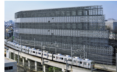
Green Hills Building No.1 2011, design Y. Tsukamoto and Nihon Sekkei, Inc.; structure T. Takeuchi; building services M. Ihara
