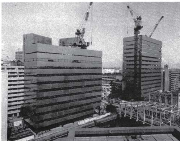
Photo. 3 No. 2 Nippon Steel Building
